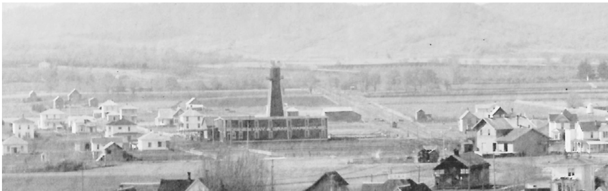
Fig. 6. The remains of the Carriage factory and its water tower; the Bodine Warehouse, ca 1907. The railroad depot is shown at the right when it was located near SW 9 th and Washington.
