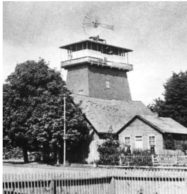
Corvallis Water Company tower located between 1 st and 2 nd street and Adams.
