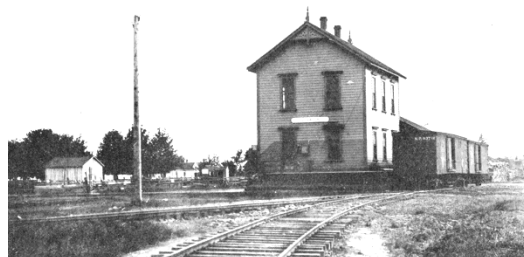
The W.O.R.R. Corvallis train depot where Irvine worked as station agent and telegrapher starting in 1880. It was located near SW 6 th St. and SW B.
