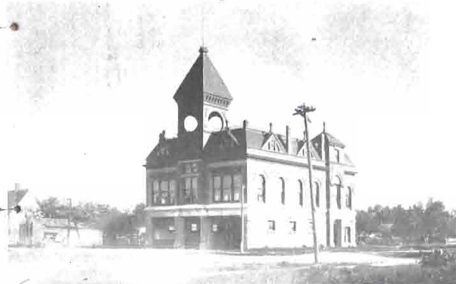
CITY HALL IN EARLY 1890'S. LIPMANN'S IS AT THIS CORNER NOW. PHOTO FROM OSU ARCHIVES.
