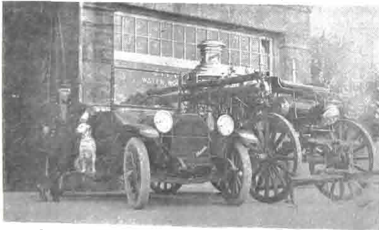
STEAM PUMPER IN FRONT OF CITY HALL. DOG IS "FRITZ." PHOTO FROM OSU ARCHIVES.
