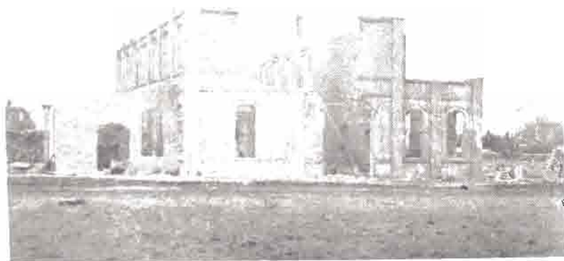
RUINS OF MECHANICAL HALL AFTER FIRE OF 1898. PHOTOGRAPHS FROM OSU ARCHIVES.
