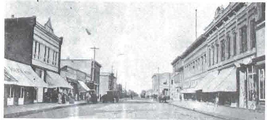
LOOKING NORTH ON SECOND STREET, ABOUT 1908. PHOTO COURTESY OF KATHERINE MCNEELY.
